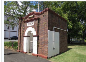
Men's Toilet, 2012, prior to its demolition in 2013 and reconstruction in 2015
